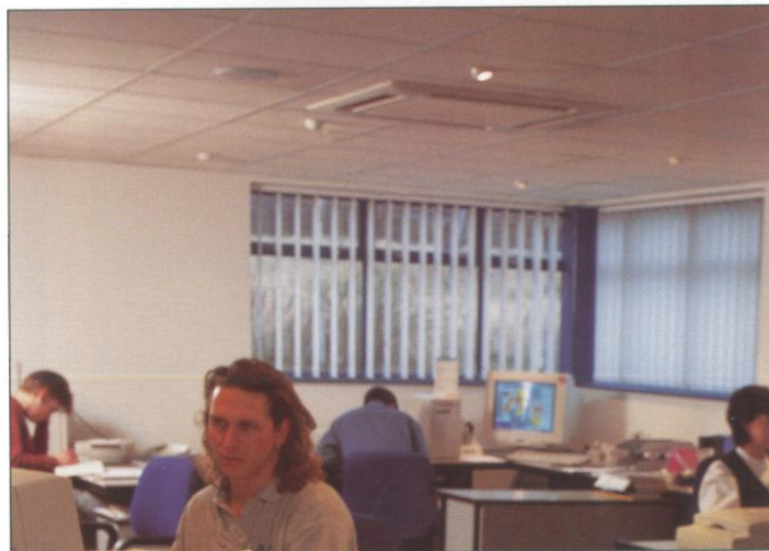
NB PRINT, WASHINGTON - Air conditioning ceiling cassettes to design studio.
