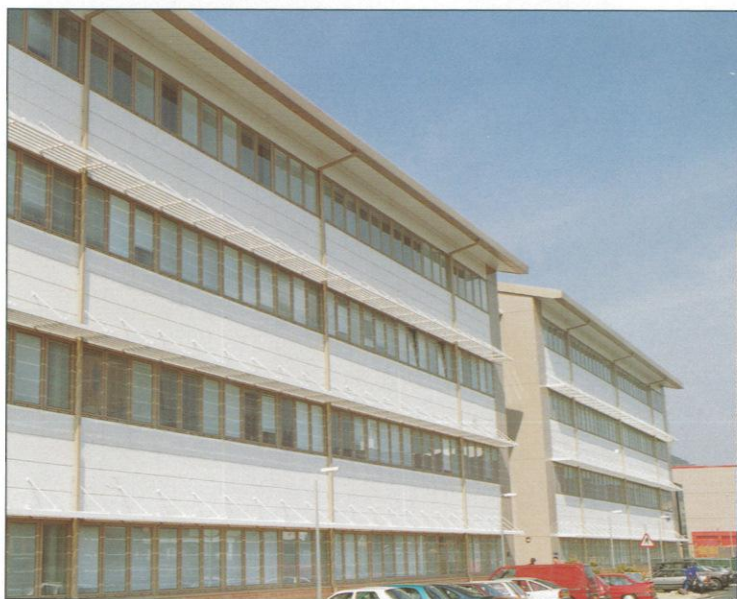
B.N.F.L., THORPE OFFICES - External solar shading. Our client: Hathaway Roofing Ltd.
