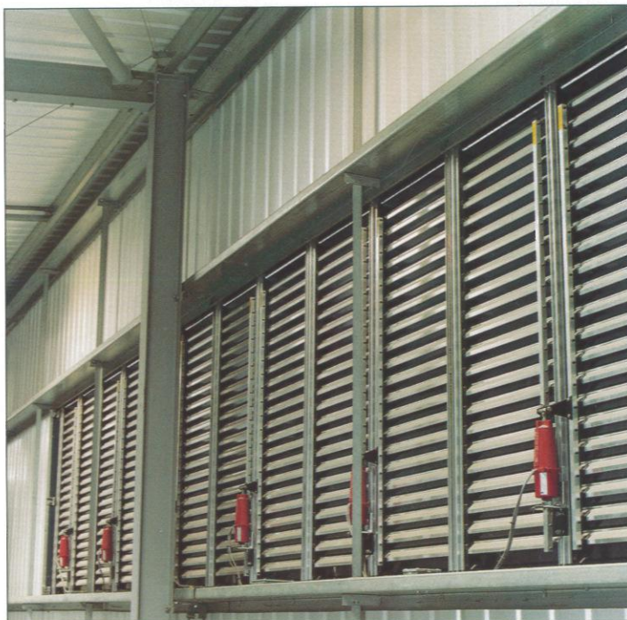
WELLSTREAM NORTH SEA, NEWCASTLE UPON TYNE - Extra performance inlet louvres with electrically operated dampers.
