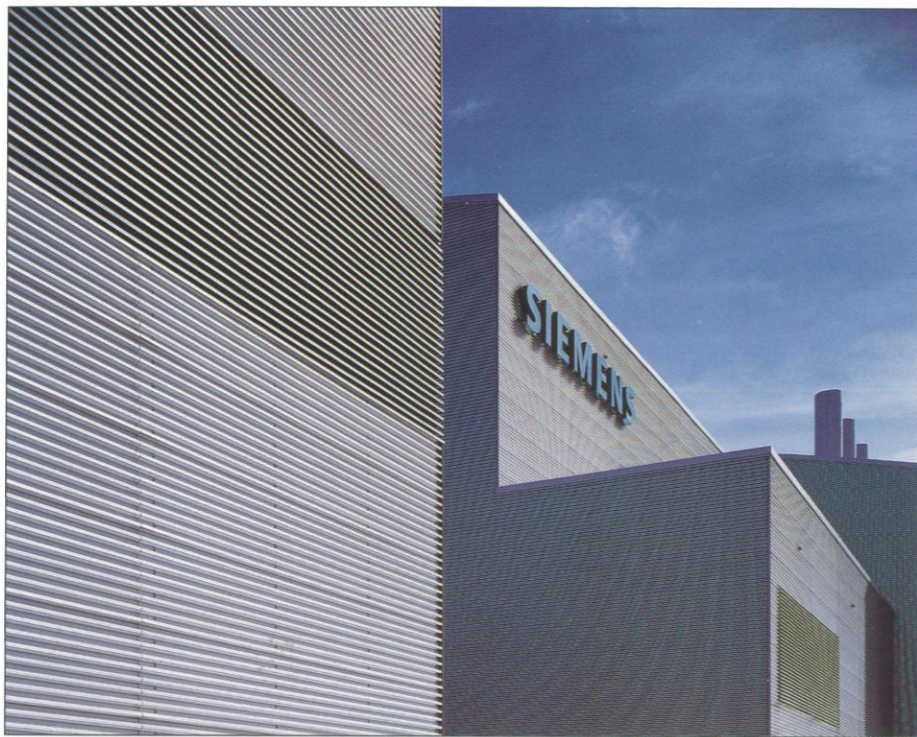
SIEMENS, NORTH TYNESIDE - Special profile louvre bank to match cladding. Architect: Parr partnership. Contractor: McAlpines/Hochtief joint venture. Our client: Hathaway Roofing Ltd.
