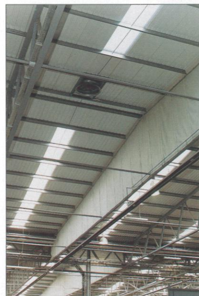
WELLSTREAM NORTH SEA - 12 fixed smoke curtains, 1 powered smoke curtain, 22 powered smoke fans with failsafe louvred smoke ventilators.
