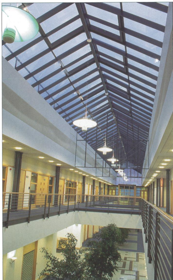
SAMSUNG TRAINING CENTRE, CLEVELAND - Glazed smoke ventilators to atrium. Our client: Kvaerner Construction.
