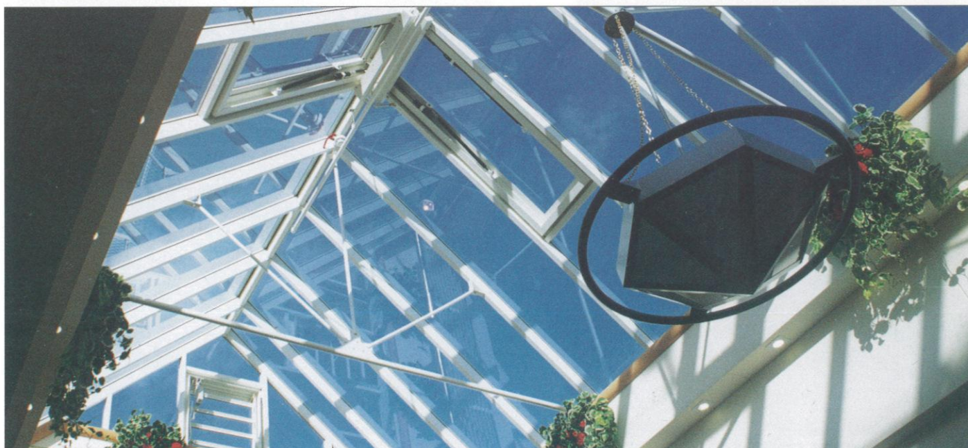
CASTLEGATE SHOPPING CENTRE, STOCKTON - Glazed smoke ventilation system. Our client: Birse Construction Ltd.
