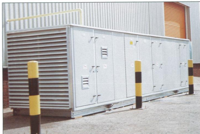
FENLAND LAUNDRIES, GRANTHAM - Gas fired air handling unit with hepa filters providing clean fresh air to clean room.
