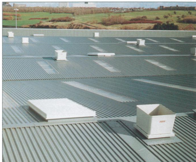
WELLSTREAM NORTH SEA - 67 louvred smoke ventilators 22 powered smoke fans 59 powered extract fans 19 adjustable inlet louvres
