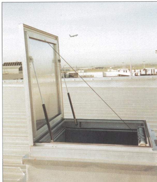
HEATHROW AIRPORT - Casement smoke ventilator with failsafe tubular motor. Our client: Hathaway Roofing Ltd.
