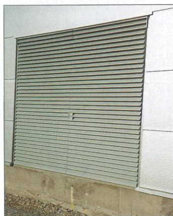
B.T. TELESales, DONCASTER - Extruded aluminium louvre panels. Architect: Stride and Treglown. Our client: Hathaway Roofing Ltd.
